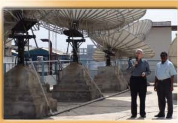
PLEDGE TODAY FOR NEW STATIONS! New TV and cable affiliate stations around the world continue to sign on every day! Just this year, TWO full power stations joined the TBN network family—including the newest, Channel 52 in Orlando! Please pledge to keep YOUR TBN strong, growing—and reaching more souls for God's Kingdom!
